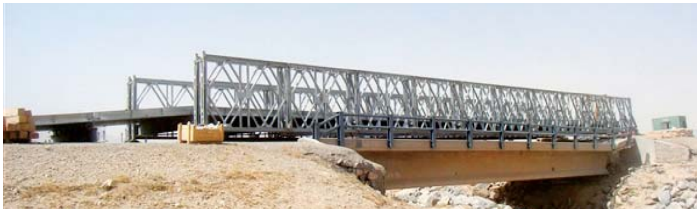
A new Mabey & Johnson Ltd. Bridge replaces a ruined bridge in Afghanistan. The Defense Supply Center Columbus, Ohio, helped get the Army spare parts for the British company’s modular bridges.
